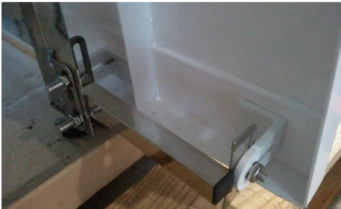
Attaching bottom brackets:
