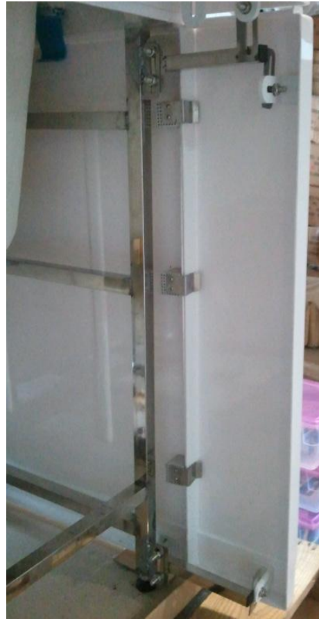
Attaching Side Panel to Skirt:
