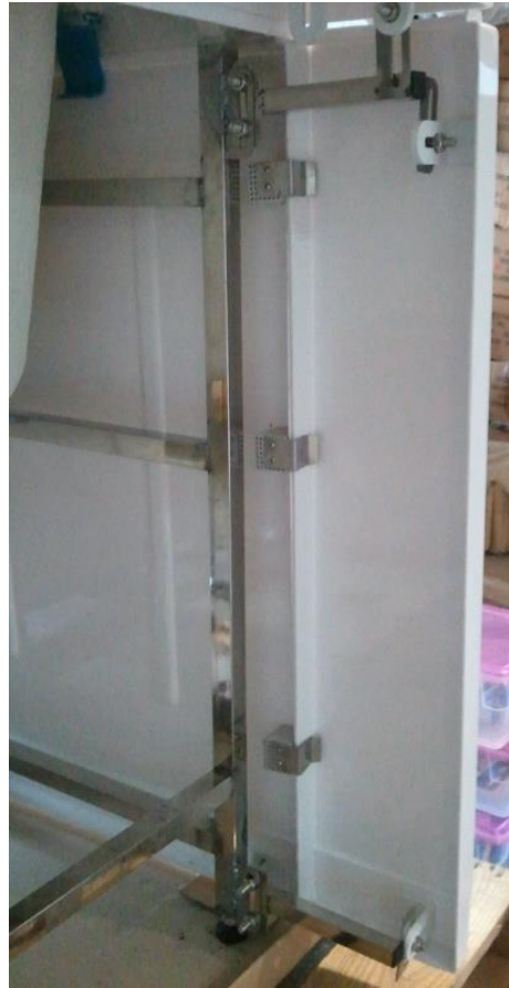
Attaching Side Panel to Skirt:
